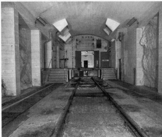
The converter station at Söderhamn in 2006. Photo by Nick Catford
